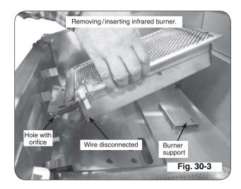
**4.** Using a <sup>1</sup>/<sub>2</sub>" <u>deep socket</u>, remove the orifice from the valve. Access this through the hole in the forward firebox plate (see PARTS LIST and Fig. 30-3).
