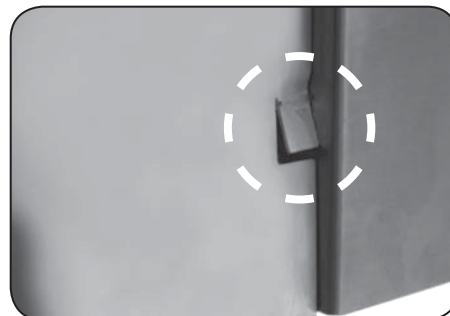
Fig. 22-2 Tab slightly bent in for clearance
