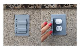
This switch/outlet combination is shown closed (left) and open (right).
